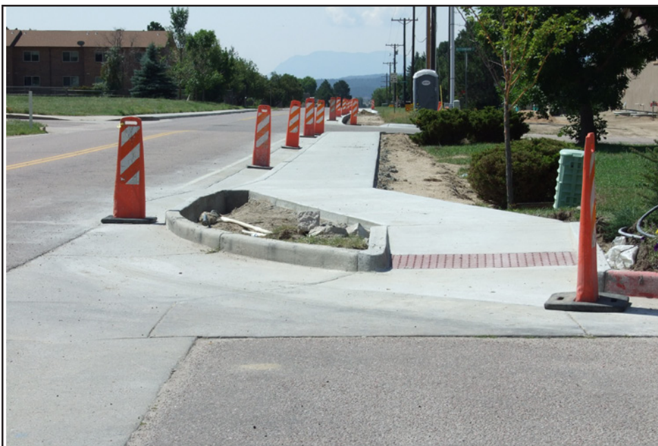
Above: Monument is getting more pedestrian-friendly sidewalks as the town installs ramps on curbs and sidewalks as required by the federal Americans with Disabilities Act. Town engineer Tom Martinez directed the project on Beacon Lite Road and Front Street on Aug. 9. The project is financed entirely by the town. Photo by John Howe.
