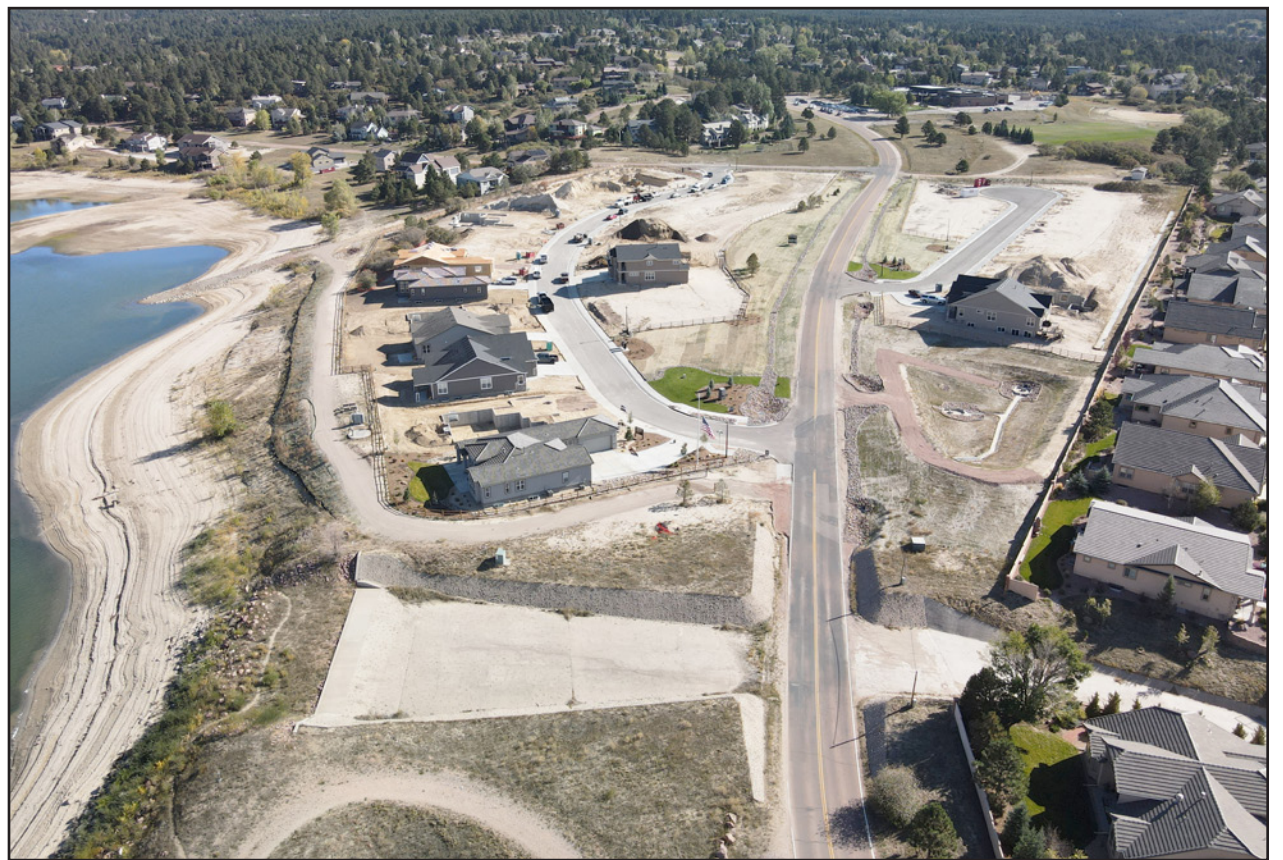
Above: Construction is proceeding at The Beach at Woodmoor, between Lake Woodmoor and Lewis-Palmer Elementary School. For more information see www.ocn.me/v17n8.htm#wia . Photo by Allen Alchian.
