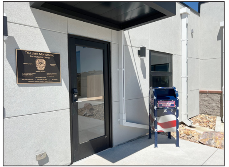
Above: TLMFPD recently installed a U.S flag retirement box at Station 1, 18650 Highway 105. The box is located at the east-facing side entry door. Photo by Natalie Barszcz.
