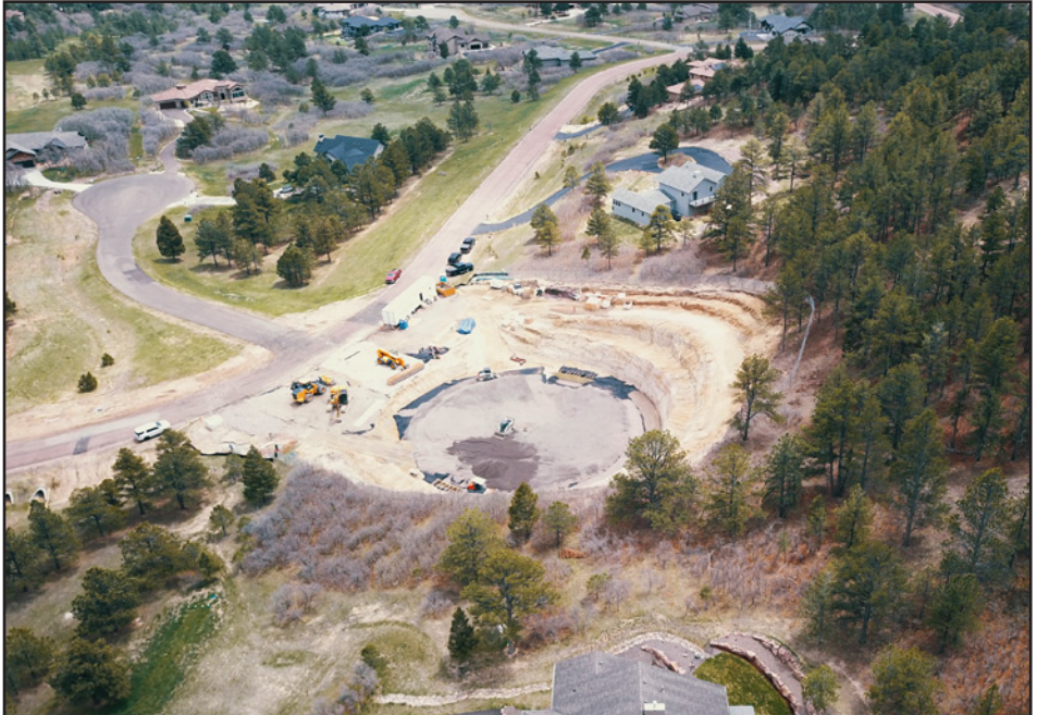
Above: On May 24, the final grade to level the base of the excavation site for the 2-million-gallon Monument water storage tank was in process to completion for pouring the concrete floor during the first week of June. This expansive storage tank project site began early in 2022. The project is closely bordered by established residential properties of Forest View Estates, adjacent to the Red Rock Ranch area. On-site pouring and casting of the concrete panels for the storage tank have already been started. Erection of the tank panels will begin later in June. Trenching for the water pipeline has already been done through the Forest View Estates and Red Rock Ranch residential roads. Continuation of laying the pipeline is progressing along Highway 105 into downtown Monument. Caption by Sharon Williams. Photo courtesy of Adams Brien.
