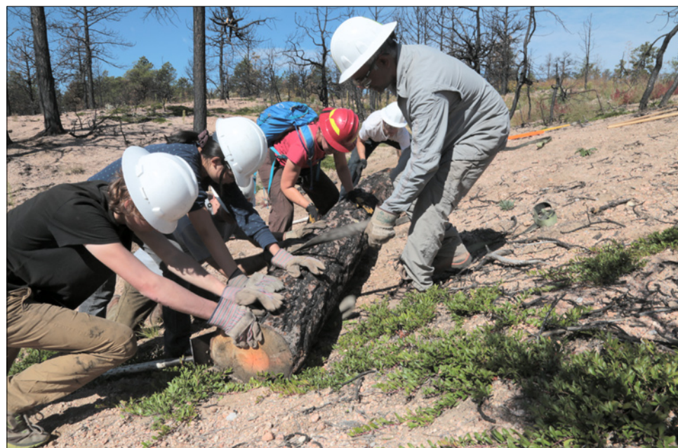
Above: The 2013 Black Forest Fire reduced the ground's ability to absorb rainwater and runoff, presenting the need for anti-erosion practices. On Sept. 13 and 14, volunteers guided by the Rocky Mountain Field Institute used pickaxes, sledgehammers, and saws to install log erosion barriers (LEBs) in Black Forest Regional Park. LEBs allow rainwater to run downhill in wide sheets instead of channeling into deep rills that erode sediment and wash it downstream, clogging drainage ditches and washing out roads. Volunteers also planted grass seed to promote slope stabilization. See www.rmfi.org for more information. See also www.blackforesttogether.org to volunteer to help Black Forest landowners with continuing cleanup work on their properties after the fire. Photo by George Lee. See additional photos on page 23.
