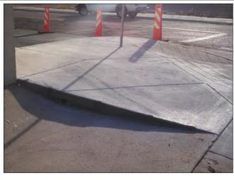
Above: The town's new sidewalk along the west side of the Monument Sanitation District building has created a tripping and icing hazard in front of the entrance to the 2nd Street Hair Salon. The town has declined to remove the problem portion of the new sidewalk and reinstall replacement concrete at the correct grade to eliminate the hazard as requested by the district. Photo by Mike Wicklund.
